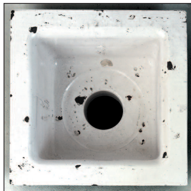
Before: This porcelain floor sink has seen better days and now is completely useless, but it can be repaired without breaking up the floor....
